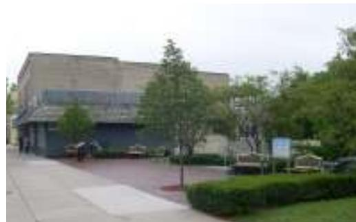
The area had become unsafe due to tree roots pushing up the sidewalk. The village removed the trees and replaced them with two new Linden trees. New cement work was completed and dyed and stamped to look like bricks. Notice also the compass stamped at the top of the stairs.
